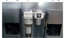
A solenoid valve adjusts the required air flow for the desired dehumidification via the device software. Manual adjustment of the compressed-air drying unit is necessary only under extreme process conditions.
